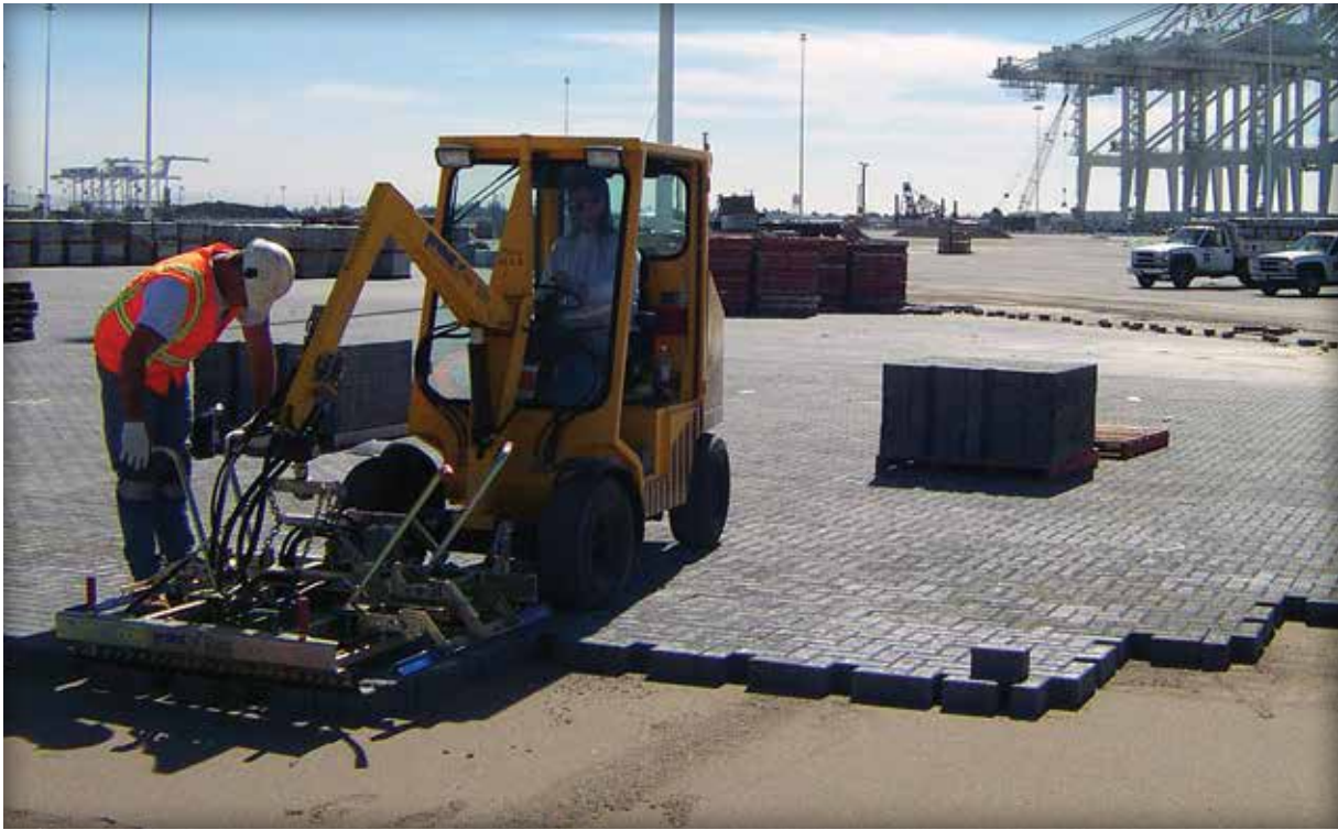
Figure 8. Mechanical installation equipment places concrete pavers rapidly.
